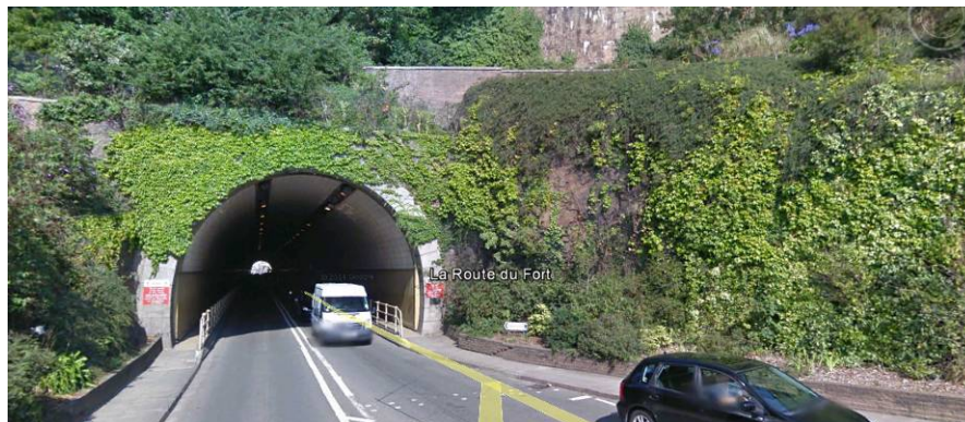
East end of Tunnel looking westbound
