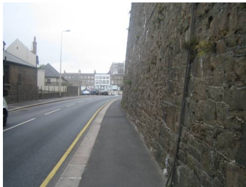
Section 8 Footway on East Side
