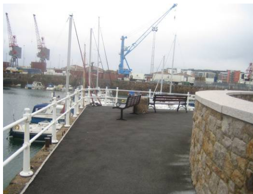
Section 10 Route between south end of Commercial Buildings and English Harbour
